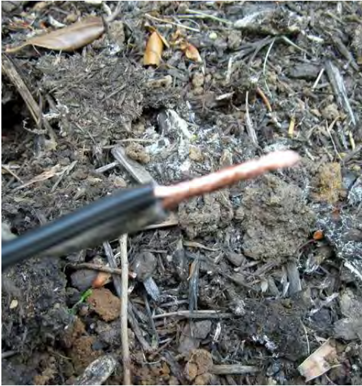
Step 1 – Strip Wire & Twist
