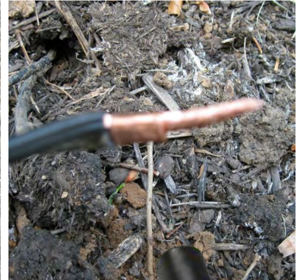
Step 2 - Crimp Copper Barrel on Wire
